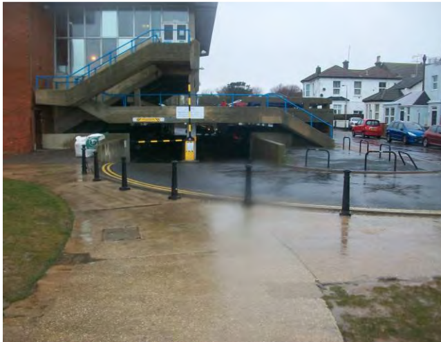
Photograph 3 – Existing Car Park Access
