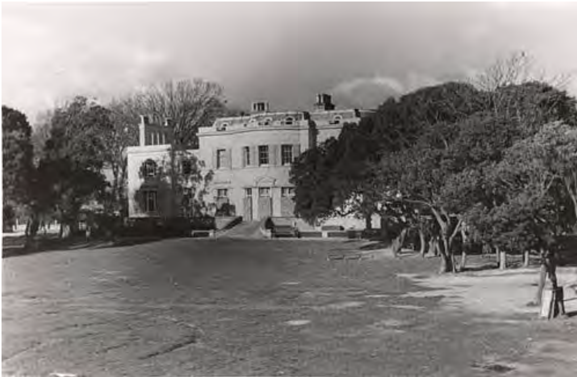
Fig.10 The south front of Beach House in 1945
