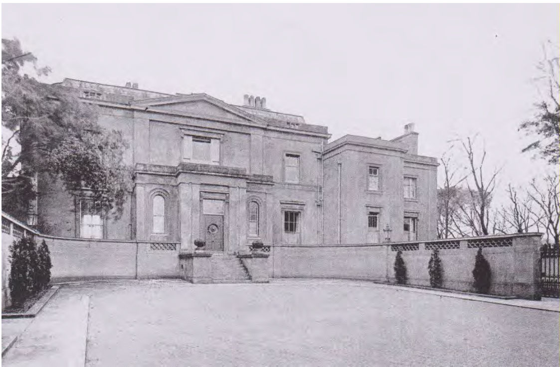
Fig.7 The north front and entrance court of Beach House in 1923
