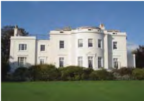
BEACH HOUSE GRADE II*
