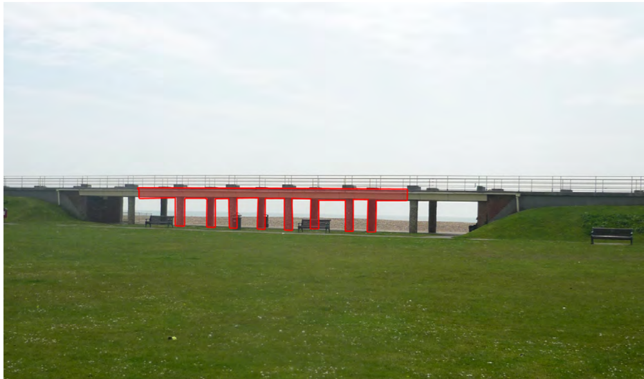
The centre portion of the raised walkway is proposed to be removed to allow increased connectivity to the beach and security for the raised terraces.
