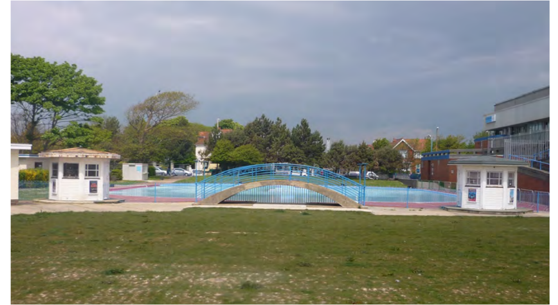
The existing splash pool and pedestrian bridge within the site boundary will be part of the demolition strategy.
