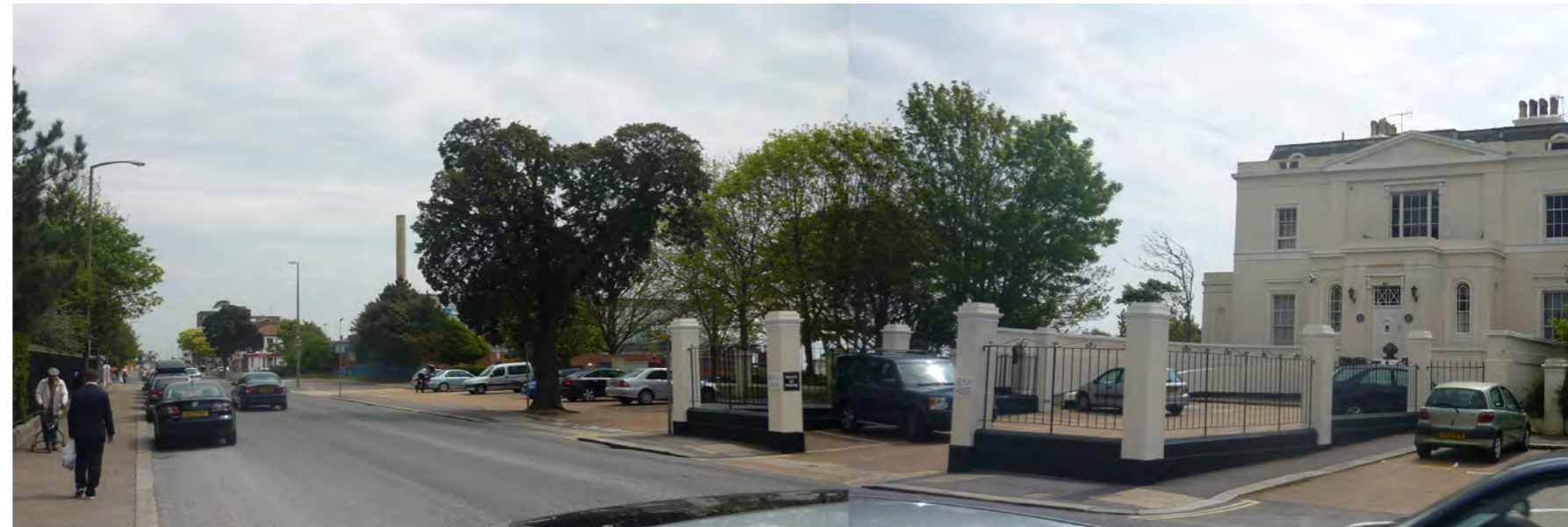
View towards Site From Brighton Road
