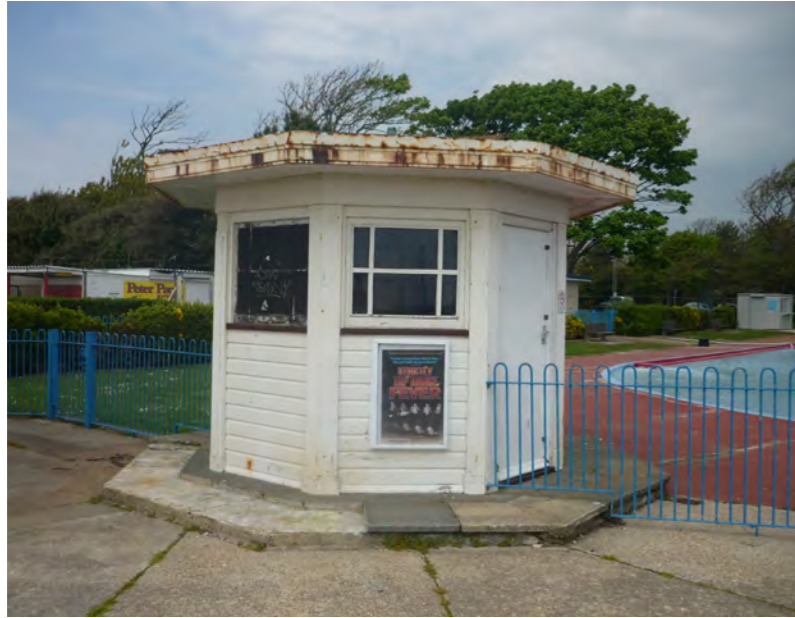
There are three kiosks within the site boundary that will be part of the demolition strategy.
