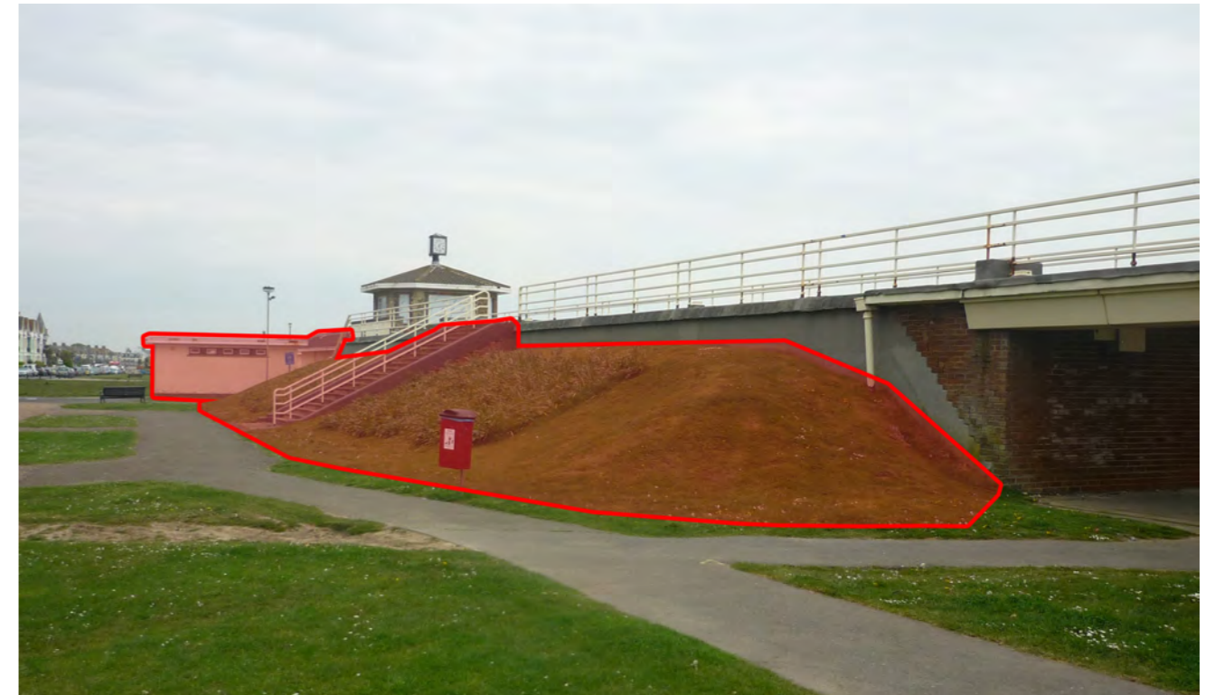
The existing landscape mound and stair access to the eastern raised walkway will be removed and incorporated into the raised terrace strategy for the proposed development.
