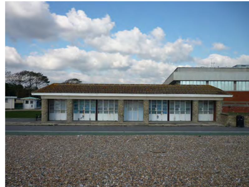
Beach Chalets to be Demolished
